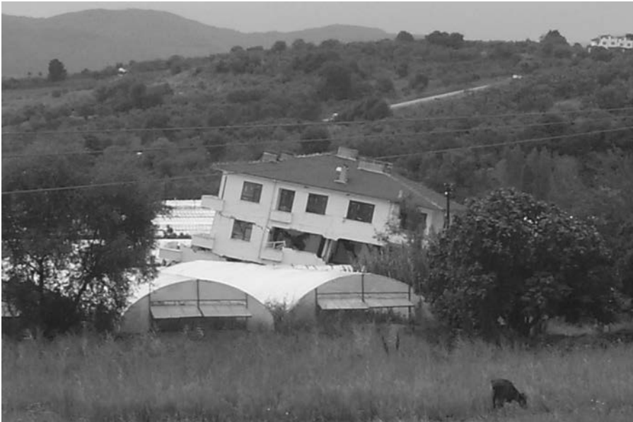
Fig. 4.1 House tilted by level-ground liquefaction in Turkey. Photo: R. Rothaus.
